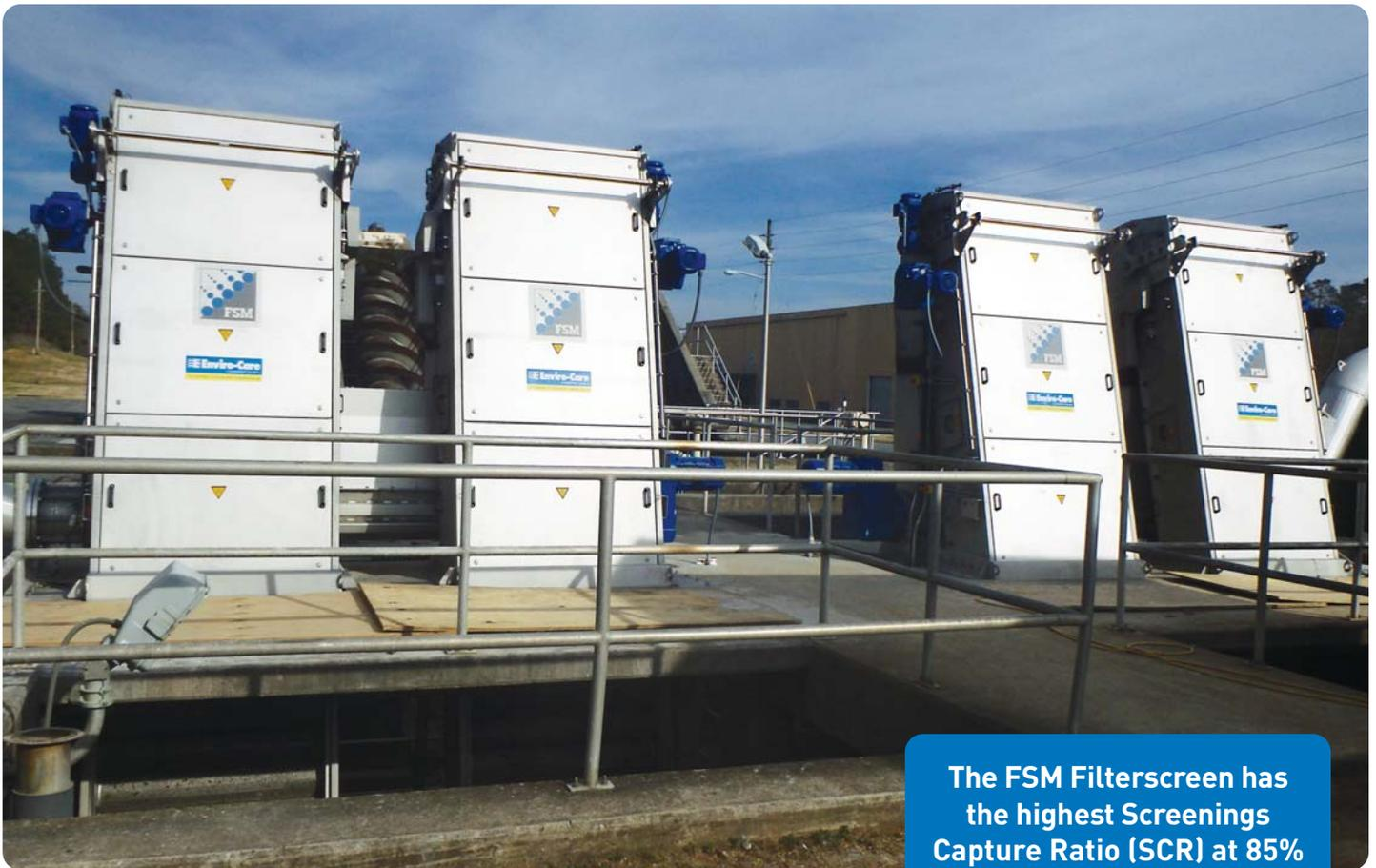
The FSM Filterscreen has the highest Screenings Capture Ratio (SCR) at 85% using 6 mm perforated media of all 59 screens independently tested at the Thompson RPM facility in the UK.
